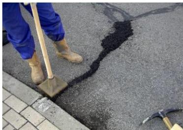
The area where **TOK®-Fill** has been installed does not need to be sanded and can take vehicle traffic immediately without further work.
