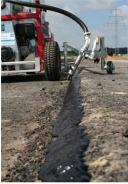
Seams in wearing courses are caused by the lane-by-lane laying of a bituminous mixture with similar properties.
